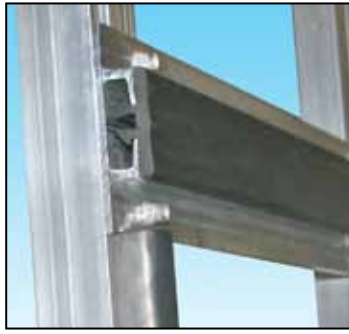
Strong 1/8-inch thick T6 aluminum posts and slats
